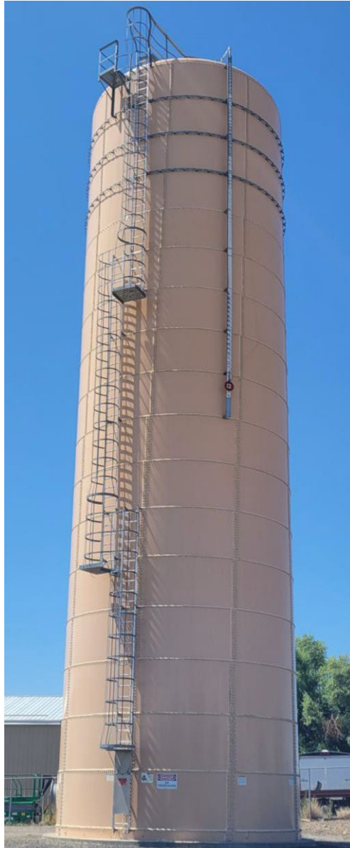
Figure 5: Glass-Coated Steel Bolted Tank Reservoir
